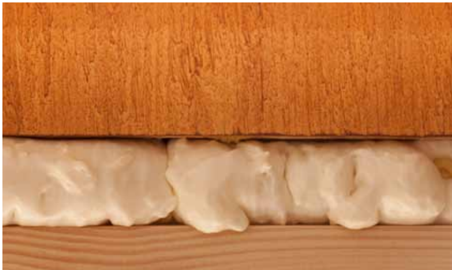
Figure 29. Polyurethane foam filling gap
